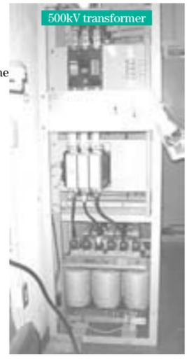
Countermeasure: Installation of transformer filter for 5th and 7th harmonics
